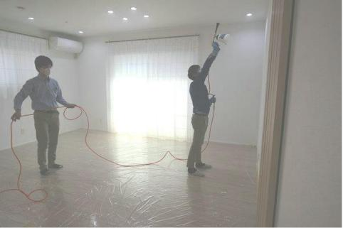
Image of photocatalytic coating service
